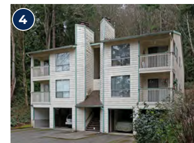
8715-8121 175TH AVE NE 8715-8121 175th Ave NE, Redmond
