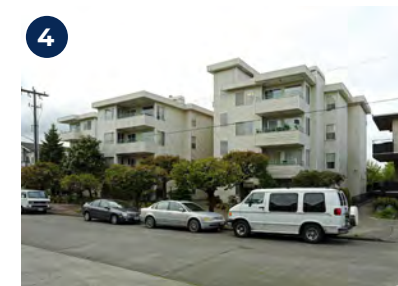
1425 NW 61ST ST 1425 NW 61st St, Seattle
