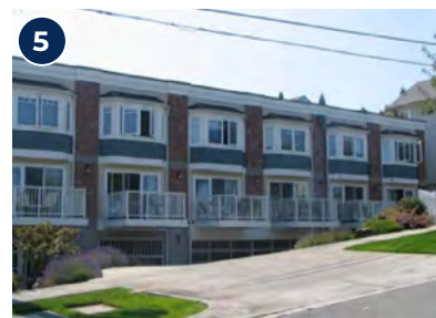
HARBOR PLACE TOWNHOMES 2406 N 31st St, Tacoma
